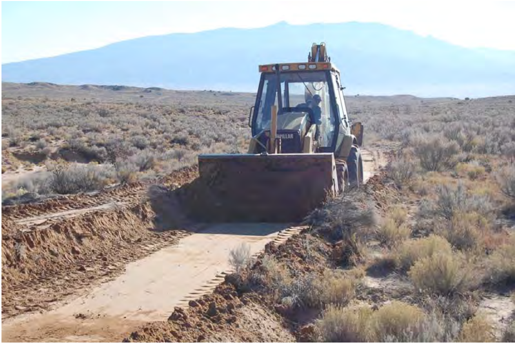
Figure 5.2. Backhoe scraping at LA 158642, view looking east.
