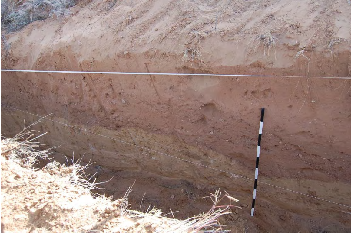
Figure 6.3. Overview of backhoe trench profile segment, view looking northeast.
